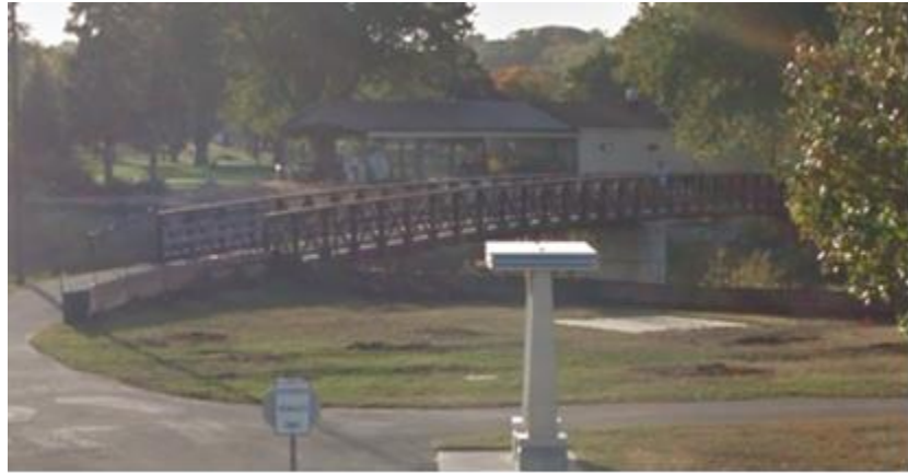
Potential Bridge for Reuse at Channel Crossing
